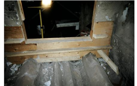
Thermbond Formula 6L formed and cast in the discharge end wall.
