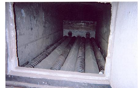
The completed repairs with floor augers replaced.
