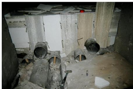
End Wall Reline with Thermbond Formula 6L in a wood waste feed furnace. Insulating board installed ready for Thermbond hot face.
