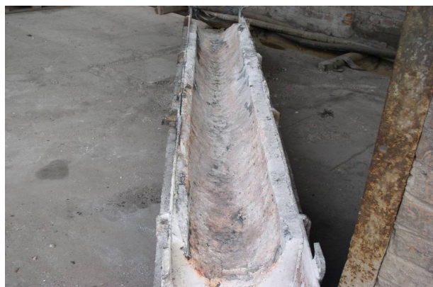
After 14 days in operation - sill in operation.
