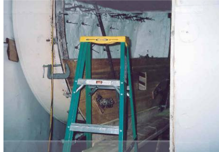
Divided into two pours - lower form in place.
