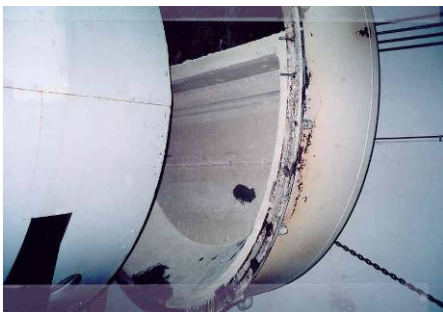
Form removed - 1 hour after pour.
